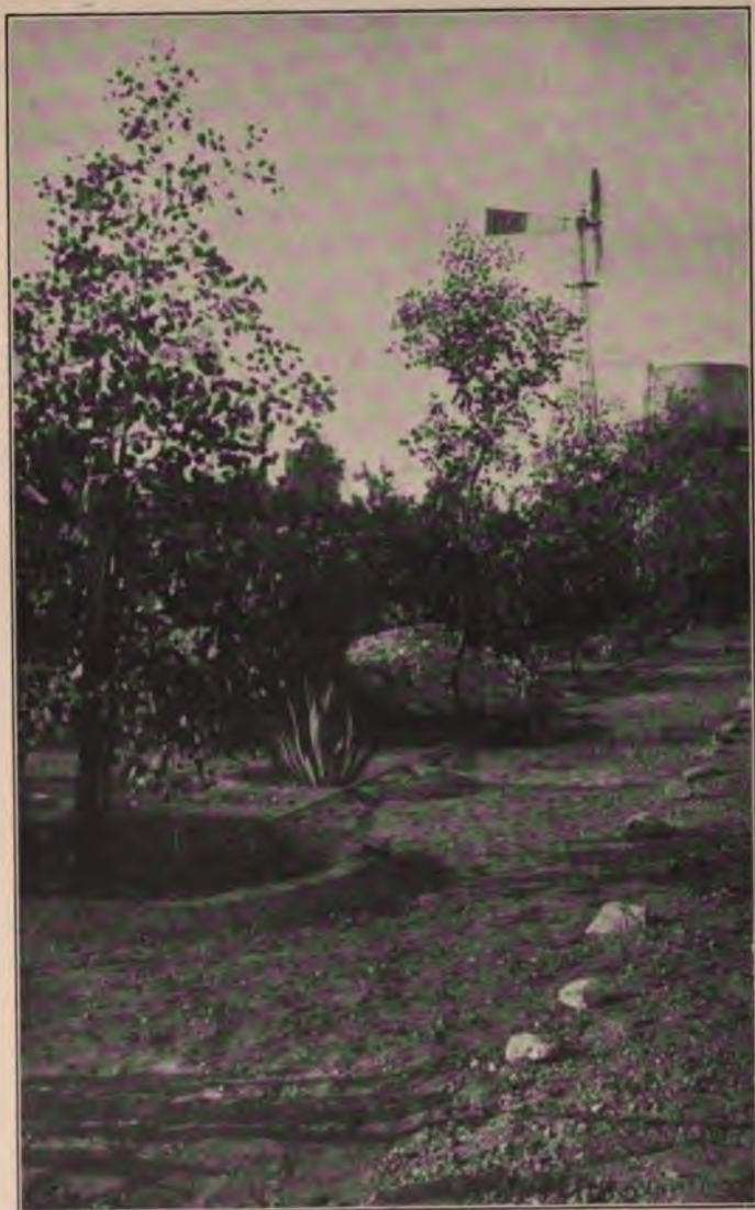
FIG. 95. Windmill and storage tank. Tucson, Arizona.
